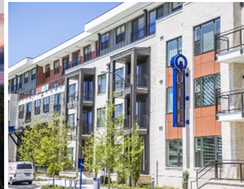
Quill Apartments at Edgewood-Candler Station
